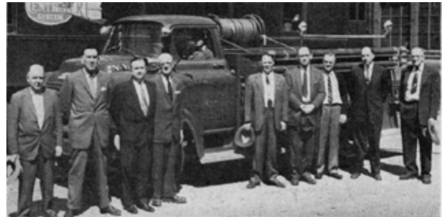
NEW FIRE TRUCK was delivered to NYC's Beech Grove, Ind., Shops while safety conference was being held there. Out to inspect the new fire fighting equipment are (from left): H. C. Briscoe, Gen. Fri. Car Foreman; F. J. Kossuth, Supt. of Car Maintenance (New York); O. L. Easton, Gen. Supt. Shops; R. B. McDaniel, Safety & Fire Protection Engineer; L. W. Black, Asst. Fire Chief (in truck); G. M. Schmidbauer, Supt. Car Shops; C. Stevenson, Gen. Passgr. Car Foreman; F. P. Neesley, Supt. Diesel Shop; G. M. Beischer, Master Mechanic of the Central's Southern District; and F. E. Kissel, Gen. Foreman—Locomotive.
