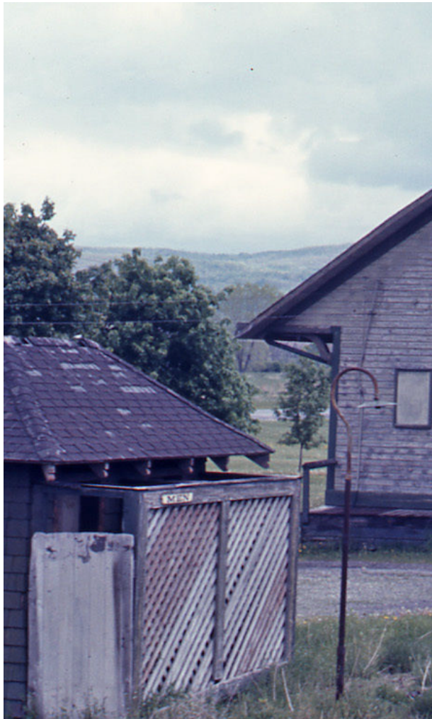
This is a photo of the Caryville Station's privy that Larry and Manuel used to help design the kit. Larry Faulkner provided photo.
