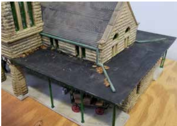
A gutter hides the canopy roof seam.
