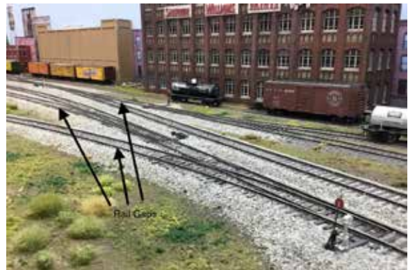
Rail Gaps to Isolate Spurs From Main.
