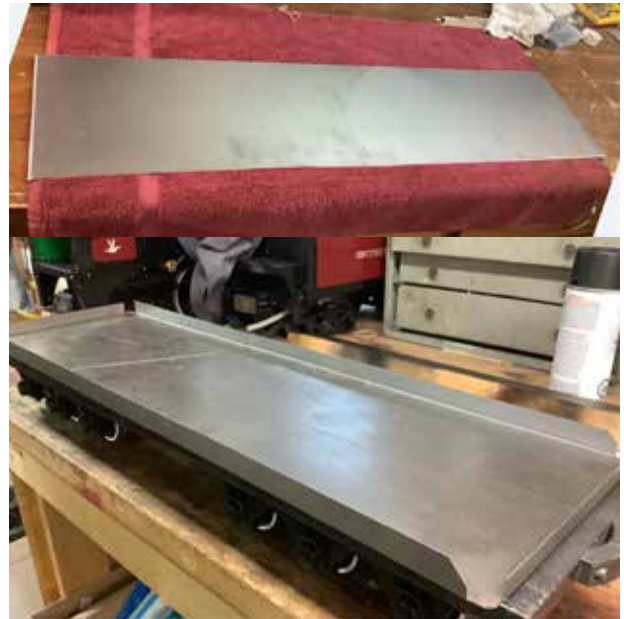
Here is a shot of the metal cut for the floor (top) and the formed metal floor (bottom) with the fabricated ears.
