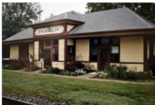
Franklin Big Four Depot (John Klinefelter Photo)
