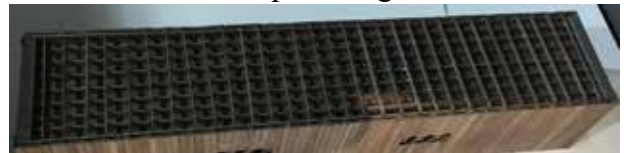
This is a view of bottom of bridge floor.
