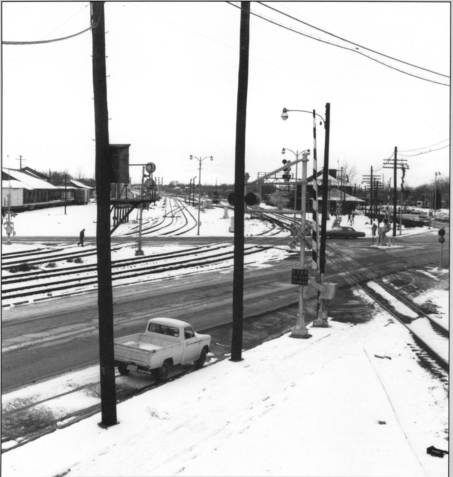
Entering Elkhart from the east, the first interlocking encountered was B, where the main line from Toledo and the Elkhart branch from Jackson converged. (Today, B is CP 421, and the line from Michigan points is called the Kalamazoo branch.) Controlled by the "Hart" operator located in the hump building, this interlocking is also the east entrance to the yard. Taken from the steps of former B tower and facing west, this photograph shows the tangent Elkhart branch and the curving Toledo mains joining just west of Main Street, with the depot a stone's throw beyond. Northern District trains from Jackson and east which used the Elkhart branch, crossed the main line to reach the two freight leads in the center of the picture. Current Kalamazoo-Elkhart trains follow the same procedure.
