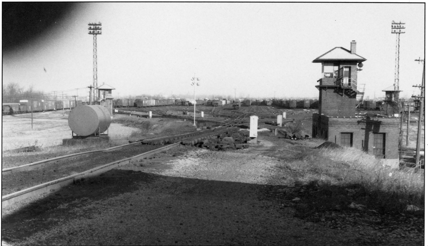
As is customary in the case of most vintage hump yards, control of retarders and class yard switches on the hump end was divided up among three sets of retarder operators (witness Selkirk, Dewitt, and Sharon; Junction Yard was an exception, having two sets). These three brick towers are in plain view here from the crest of the hump, as in the 42-track class yard, known as "K" yard. Since Stanley had no departure yard at the time, the class yard was decorated continuously with blue flags, which of course meant dead tracks and lost classification room. The consequence of this was indicated by the folly, illustrated two photos ago, of doubling out a train, only to backhaul it more than a mile to preserve switching room.
