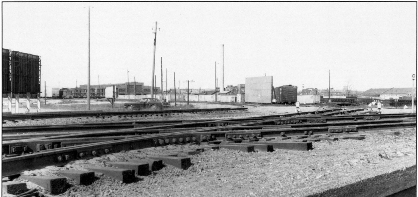
This is Waterman Avenue, the entrance to the south receiving yard from the Toledo branch and Wabash (NS) Railroad. The two Wabash tracks run across the picture in the foreground; the lead from the Toledo branch crosses them on the diamonds, and the connection from the Wabash curves around on the left. A TV camera here saw car numbers for the clerks at Livernols Avenue on such entrants as MC-2, LS-5, TB-10, River Rouge liners, and Wabash cuts. Arrivals from the West such as ND-4, ED-2, and extras from Jackson enter from the opposite (hump) end of the yard and did not get TV coverage. Departures from the south receiving yard at this end included interchange runs to the C&O and Wabash and occasionally liners to River Rouge (which more often departed the Junction Yard branch). The Flexivan pad is visible in the background.
