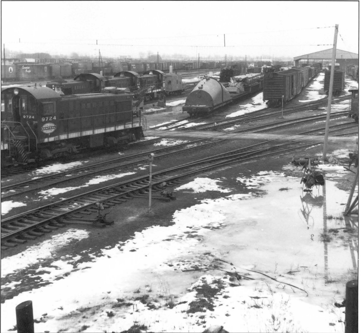
The E-L embankment on the opposite side of the YMCA building affords a good look at the car repair and transfer tracks. Four tracks, three of them for production, pass under the shed. The cycle on cripples is that they are humped into track 20, then pulled down and shoved toward the shed, where they are worked through the A-frames from west to east and moved by rubber-tired crane into track 19, from which point the humper pulls them back as "OKs" to be rehumped. The odd-shaped tank, tractor, and poles on the open-top cars identify Car Shop track 5, on which transfer and adjust loads are worked by mobile crane. The cars in the background are in Groups 4, 5, and 6 in the class yard, and again, the loop tracks are in front.
