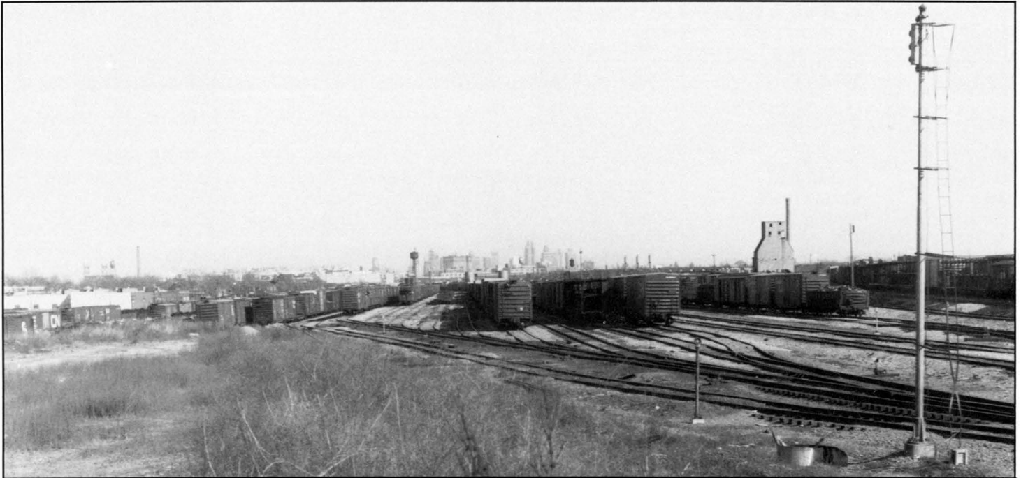
From the west end of the eastbound class yard looking east, the Livernols yardmaster's tower from which the two previous pictures were taken is barely recognizable in line with the water tower just to the left of the tall buildings in downtown Detroit. In the left background is the Glory yard, from which the most southerly track, number 11, extends along the eastbound class ladder in the foreground. From left to right, tracks 1 through 10, except 2, run off this ladder, then continuing to the right are the "Boulevard," 24, 25, and 26 (the first customs track, with a car of scrap west out). On the far right, at a higher elevation, is the south receiving yard. Though both the eastbound class and north receiving yards are in line with the hump, they were used as departure yards for transfers ("Liners," per old MC terminology) to terminal points such as North Yard, Mound Road, and Windsor. Cars for these runs were pulled back either over the hump or (from tracks 2 through 5 in the class yard) over a running track just north of the hump.
