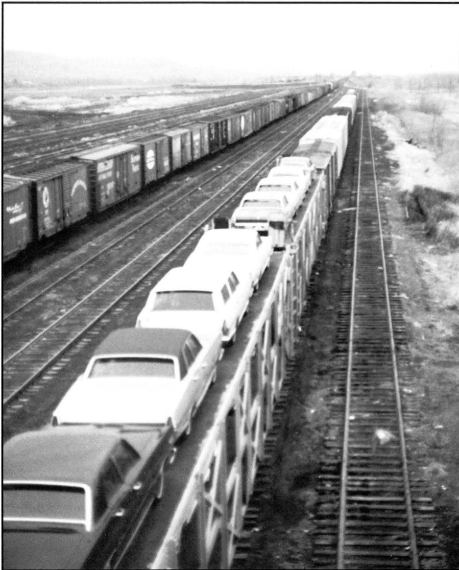
Mosher Highway overpassed Selkirk receiving yard at about its middle and from this vantage point looking west towards the hump, we see cuts to be switched on tracks 14 (foreground) and 10. Through use of track 10 and the lead extending to SK, the maximum of approximately 135 cars could be yarded without blocking other tracks. BV-3 from Boston in the instant case filled up this slot. The hump crest and hump office building are visible in the distance. Photo by J. Taylor.
