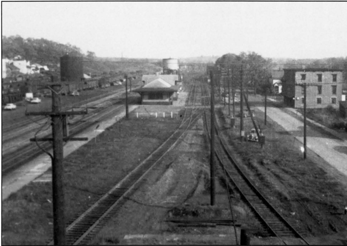
Looking east from Tower 15, towards the Lyons station. The main line passes to the left of this building. The Pennsylvania Division connection is the first track to the right of the station, and the West Shore connection comes in from the bottom right. Note the water tank east of the station, and the Iroquois Hotel, the boxy building to the right. Photo by D. M. Cosgrove.
