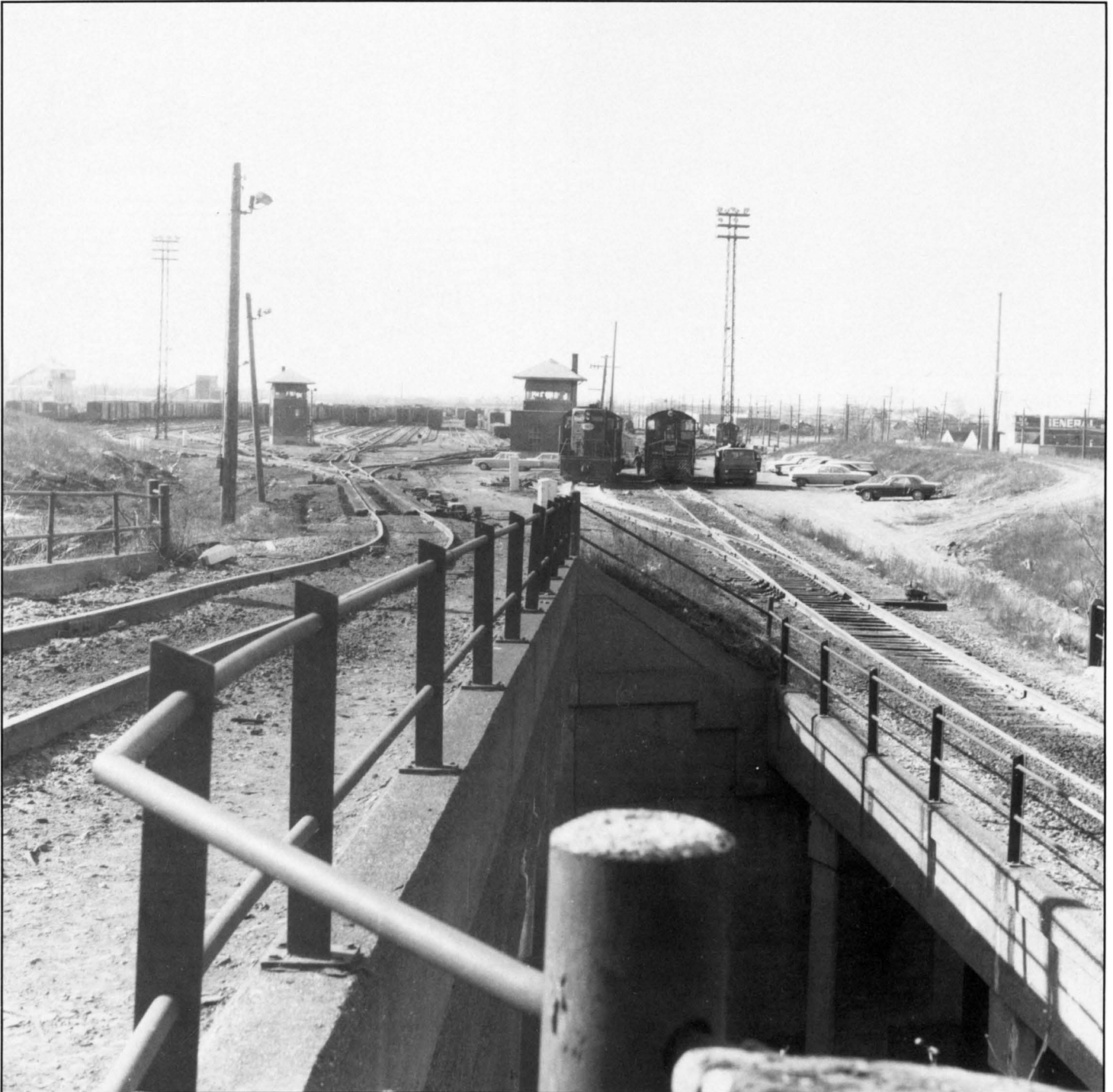
Retarder towers A and B sit astride the entrance to the 31-track class yard. Tower A in the foreground, in addition to housing the retarder operator and his control apparatus, provided office space for the hump yardmaster. The hump lead on the left and the running track on the right between class tracks 2 through 5 and the Glory yard overpass Lonyo Road at this point. Lonyo Road and Central Avenue, which intersect Junction Yard at its midsection and which are extensively bridged, provided headaches for planners trying to work out a reasonably economical plan for improvement of the yard. Surprisingly, the main tracks (behind the fill on the right) cross both of these streets at grade.
