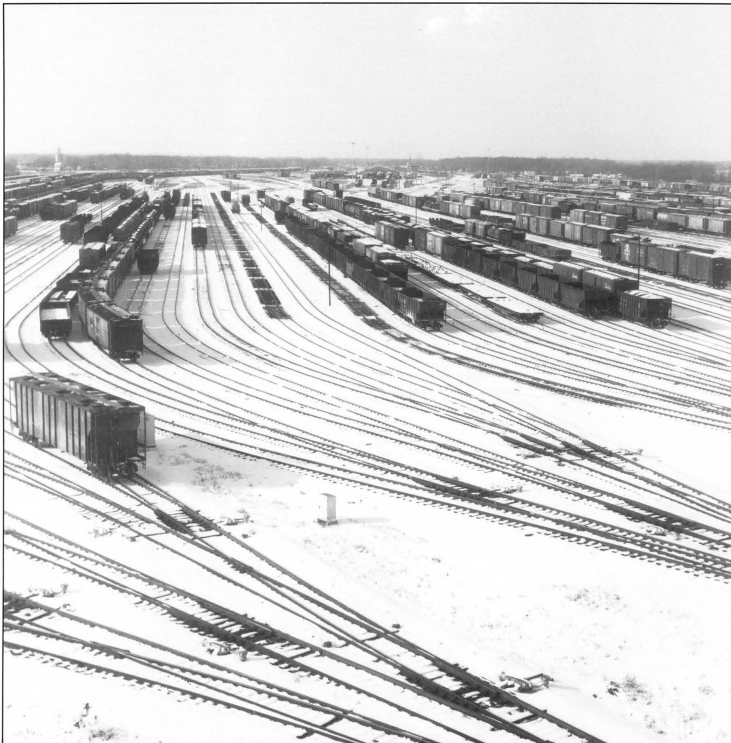
This is part of the view the retarder operator has from his post on the sixth floor of the retarder building. (Except for maintainers, he is all by himself; the trainmaster, hump yardmaster and clerical forces are all located in the hump building.) Group 7 is straight ahead, and beyond it are outbound trains in the westbound departure yard. The car shop shed is in the center background, and just to its right is the west end yard office building. Cars on the extreme right are in the eastbound departure yard, and the line of boxcars in the far left background are on the south cleanout track.
