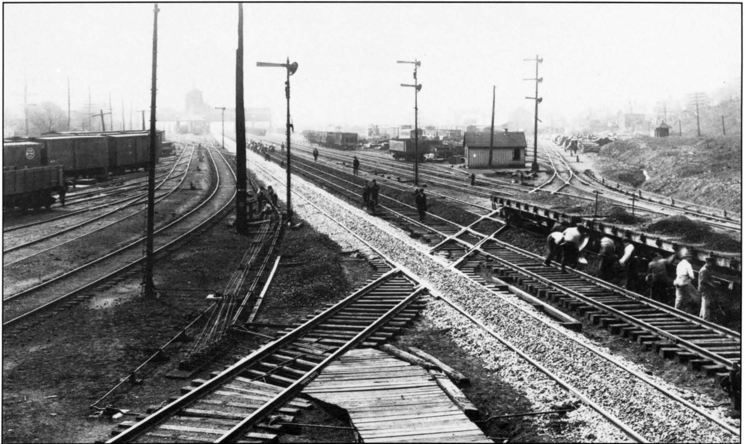
This scene is from Tower 14 at the east end of Lyons in 1912. Note that the switches are rod-operated and the signals cable-operated. The yard on the left is for the Fall Brook line, whose main tracks are between this yard and the main line. To the right of the main line is the North Yard. In the distance is a six-track coaling plant, the existence of which Mr. Cosgrove first learned from this photograph. Photo from D. M. Cosgrove.
