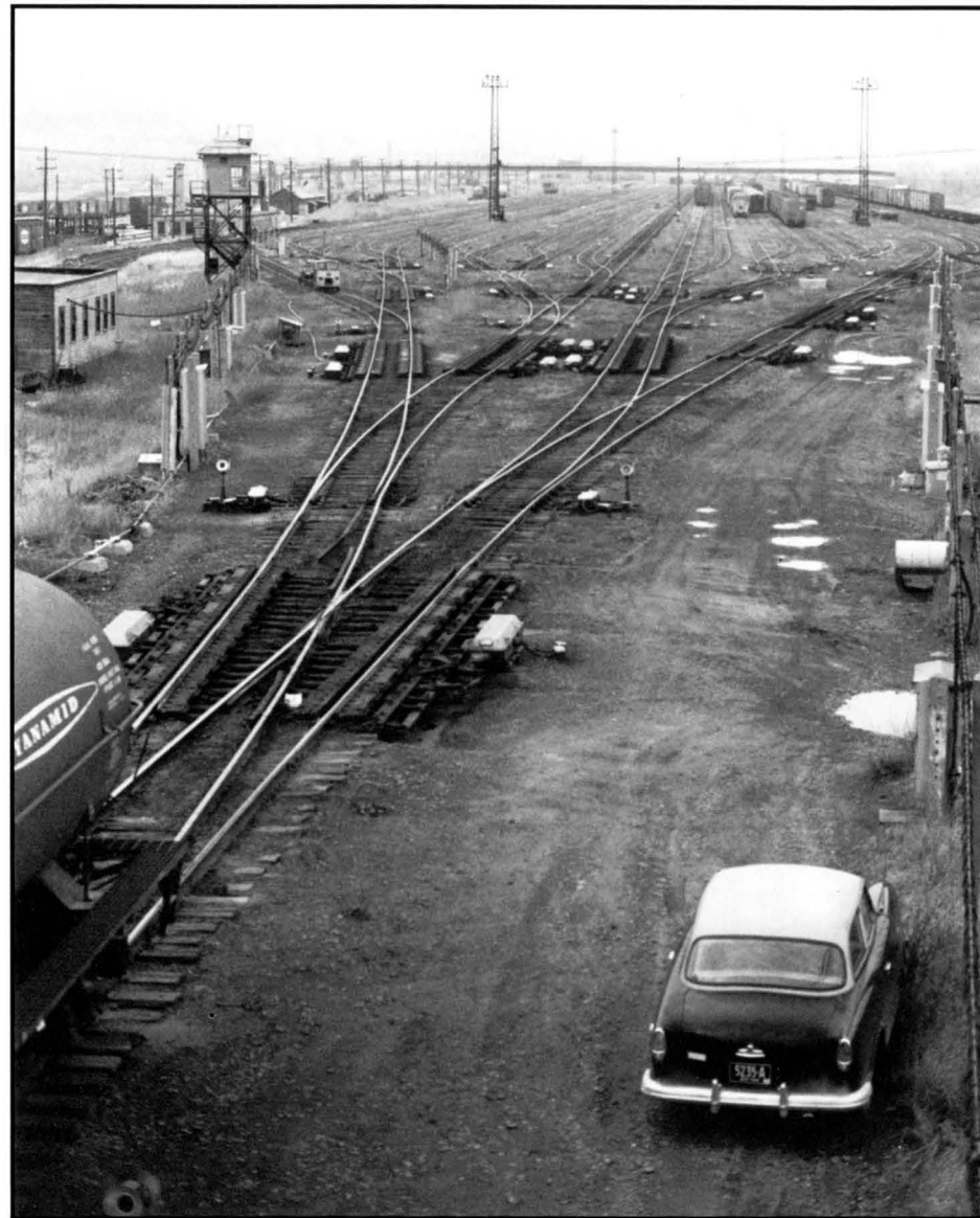
From retarder tower "A" near the foot of the hump, we look out towards the class yard, flanked by towers "B" on the right and "C" on the left. The operator in "A" controlled the retarder in the foreground and others between it and the hump crest, as well as the three divide switches in the foreground. Operators in "B" and "C" split up the balance, the former handling the even-numbered side and the latter the odd numbers. Tracks 10, right, and 8, left, run down the middle. The car shop is on the left behind tower "C", and Jericho Road bridge is in the background. Photo by J. Taylor.
