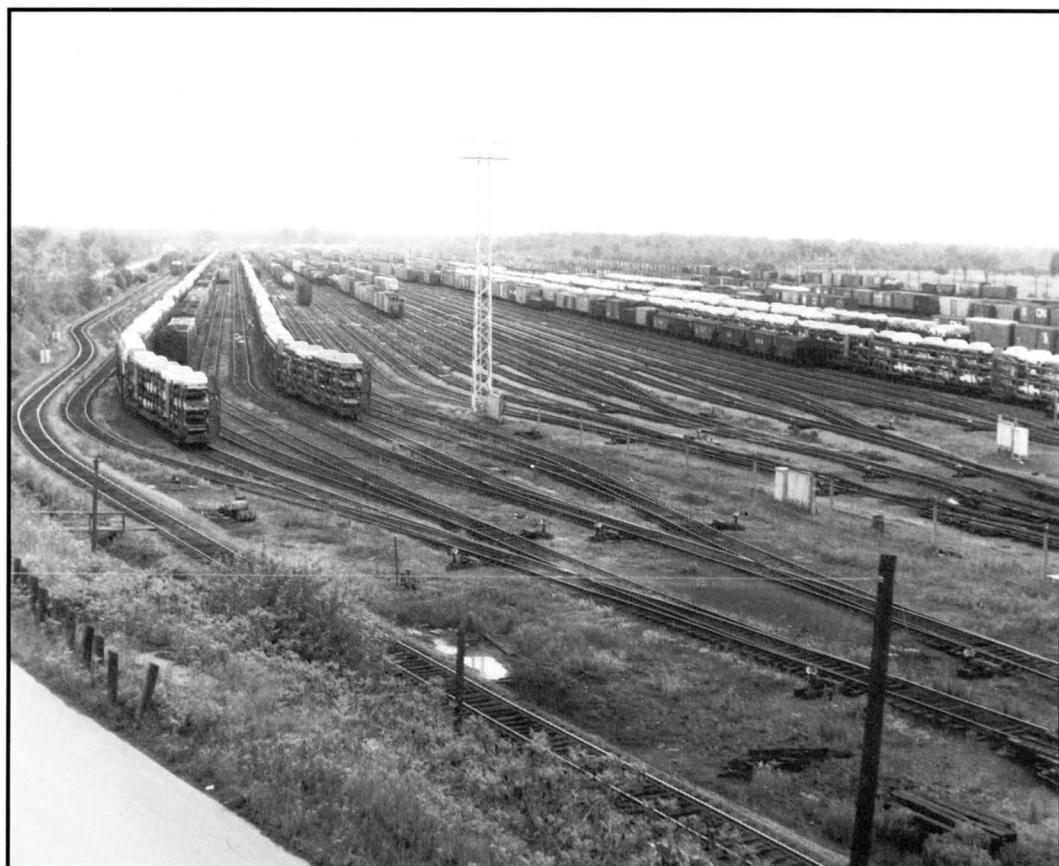
Loaded multilevels from a very late ML-12 dominate this view of the eastbound classification and departure portion of Dewitt. (At the time this was taken, the function of humping ML-12 had been shifted from Selkirk, due to advanced construction activity and resulting further emasculation of the old yard at that point). Selkirk and Little Ferry groups identify tracks 39 and 47 on the left, while Framingham autos occupy tracks in the Eastbound Class Yard on the right. The long tracks of North Yard which extended through to the east end at Minoa begin with number 19 (the eighth track to the right of the light tower). In the foreground is the engine running track between the diesel facility and Minoa. Photo by J. Taylor.
