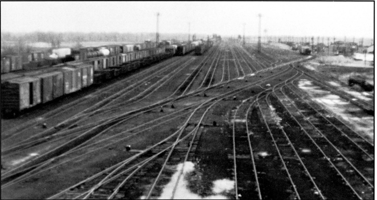
The dual ladder at the west end of class yard track 22 thru 8 (even numbers) and 7 thru 31 (excluding 27, odd numbers) was paralleled by the ladders at the east end of the "MDI" (for Merchants Dispatch Incorporated) and reclassification yards. In addition, this view east from Jericho Road bridge includes the car shop, right background, and hump, center background. That the bulk of classification work at Selkirk was then confined to second and third tricks is evident from the clear tracks and lack of activity. Photo by W. M. Gardiner.
