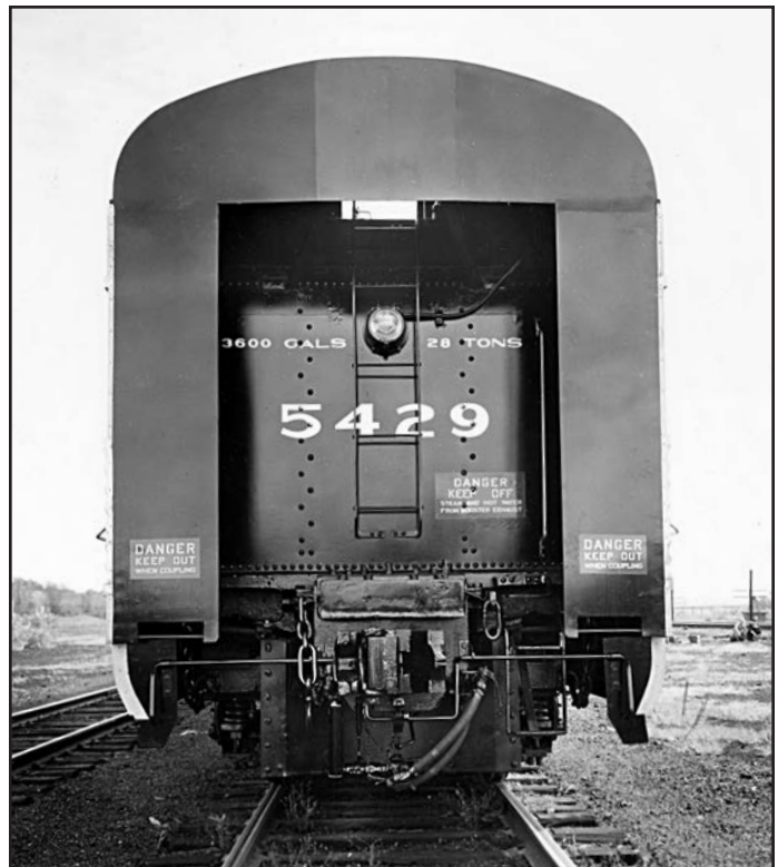
The details of the extended shrouding of the 5429's tender are depicted nicely in this second company photograph of the streamlined locomotive, taken on the same October 10 day. NYC Negative 5978-1, NYCSHS Collection.
