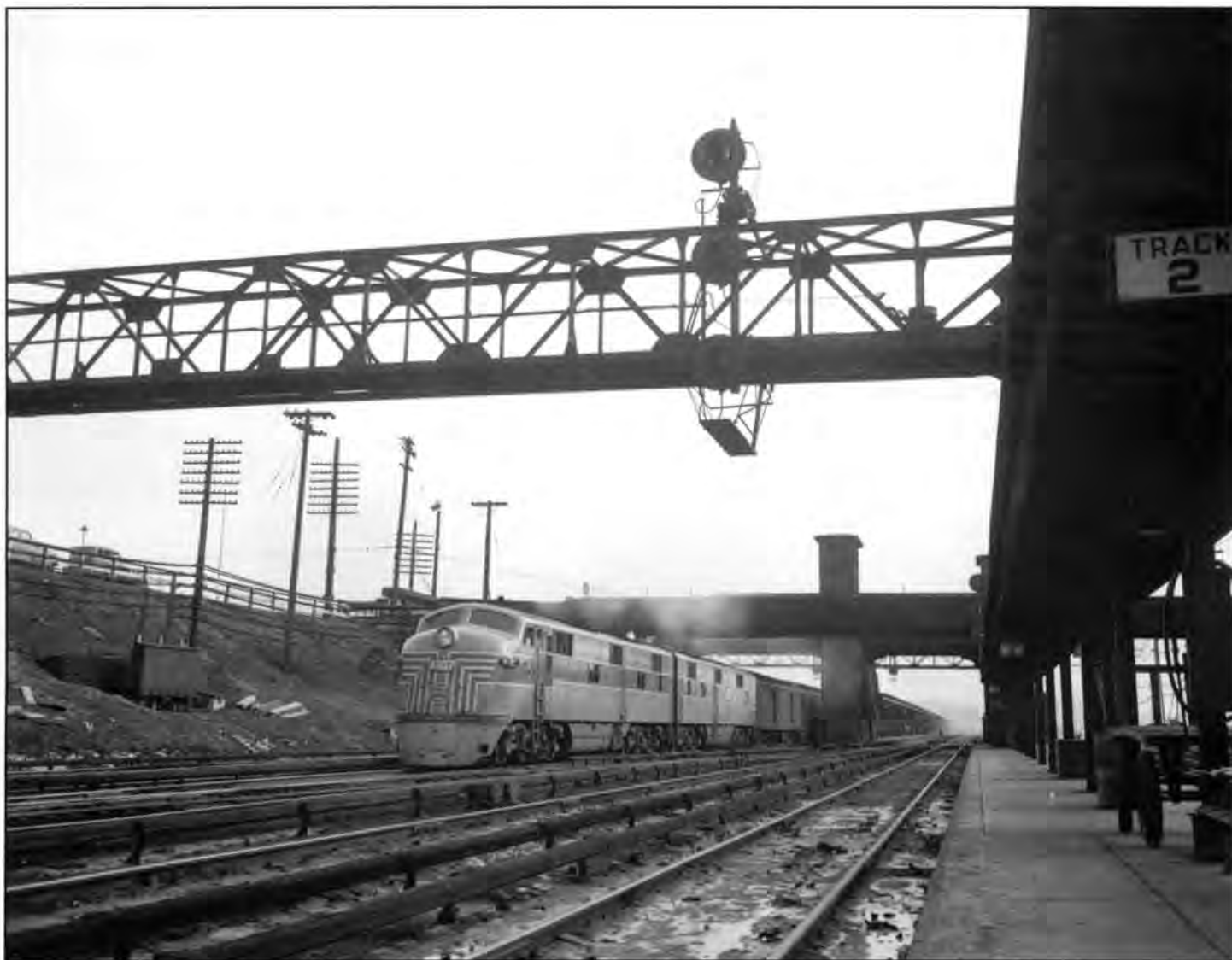
The electric has cut off, and 4007 heads west with her train. Train consist may indicate a secondary assignment. Negative 7200-3.
