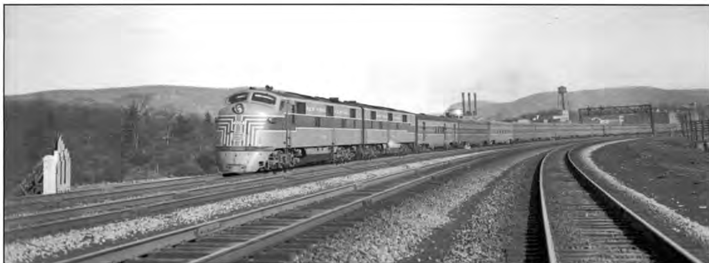
E7 4004 with Eastbound #26 traverses Fleischmann's Curve at MP 40, Peekskill, NY, on April 7, 1946. Negative 7240-1.
