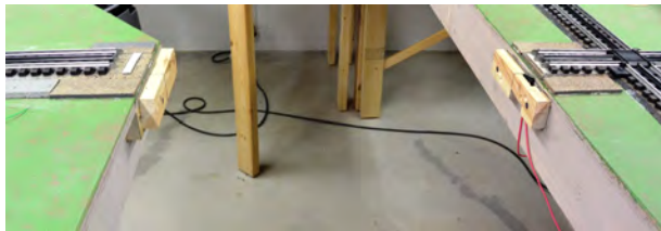
The lift-out bridge spans a 22-inch aisle, and rests on mounting blocks affixed to horizontal bench work rails on each side of the aisle.
