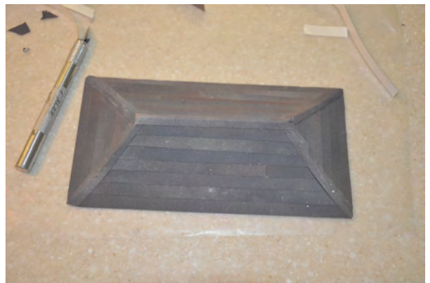
The rolled roofing strips are glued in place starting at the bottom of the roof and working up to the top. Once all of them are in place, folded panels are used to replicate the flashing strips along the rooflines.
