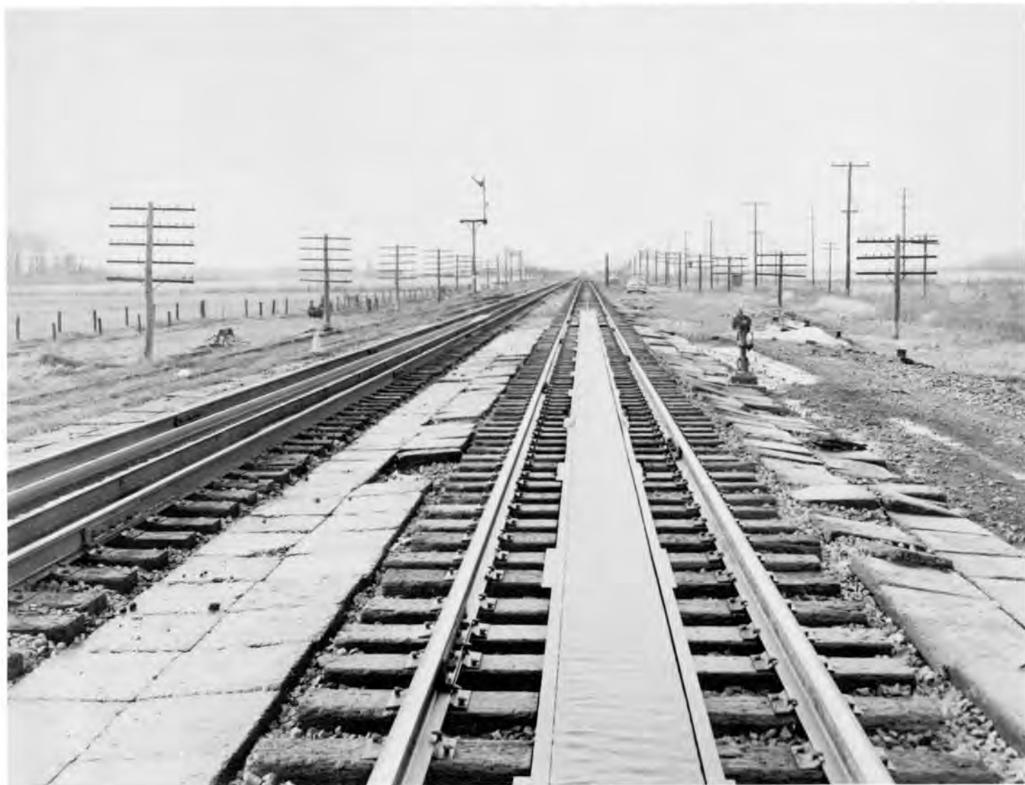
Looking west towards end of Lydick, Indiana track pans, Track #1, November 20, 1945. Purple indicator light for end of pan at right. NYCSHS
