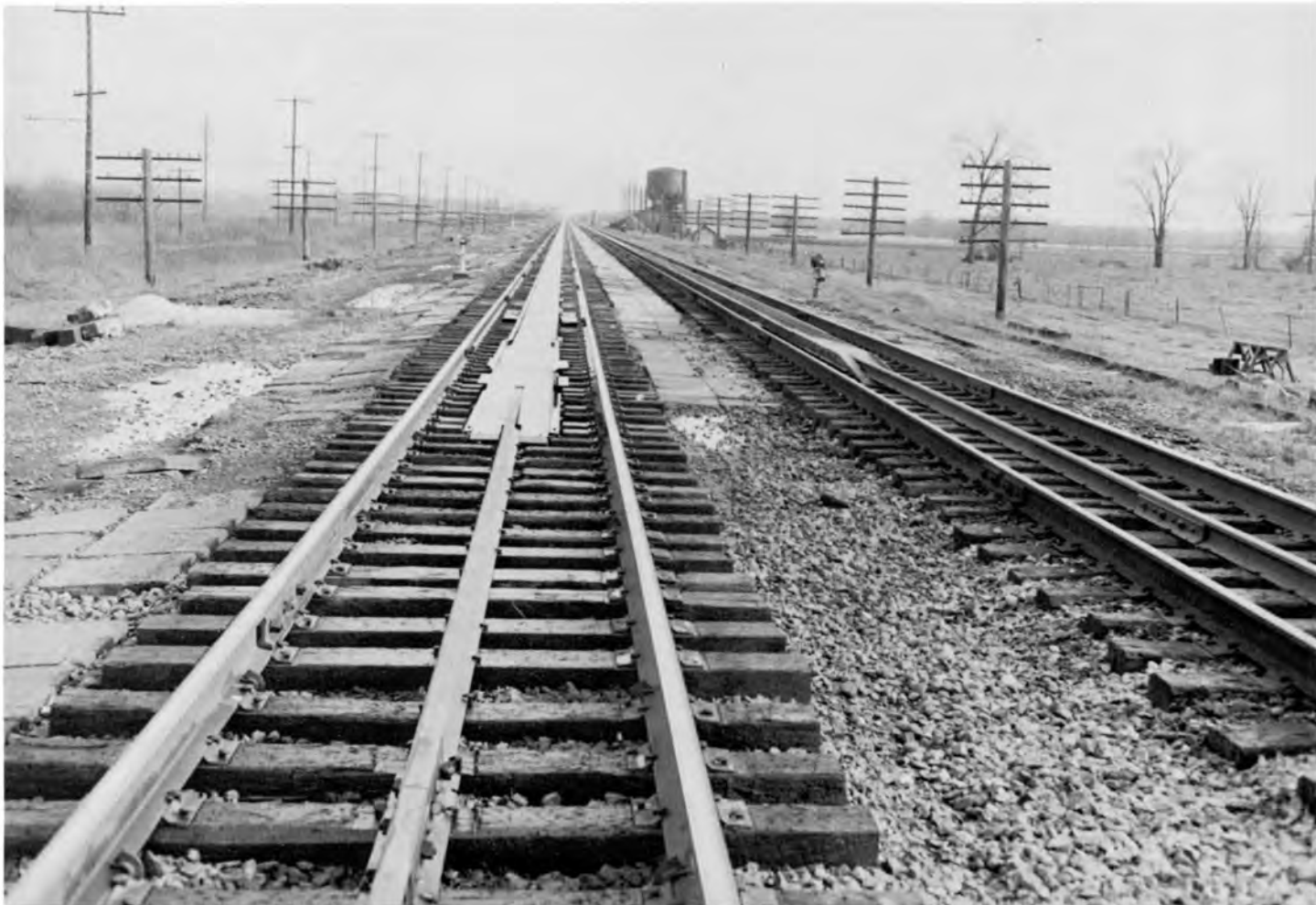
Looking east at Lydick, Indiana track pans, Track #1, November 20, 1945. Note the guard rail at the end of pan. NYCSHS
