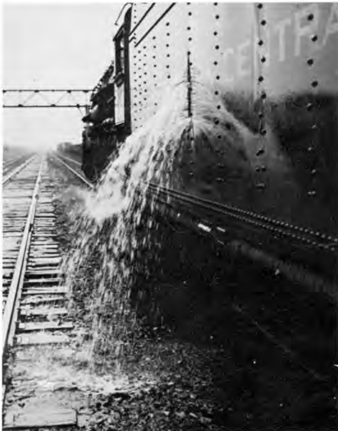
Before vents were installed, pressure built up and cracked the side of tender while testing the new design scoop.
