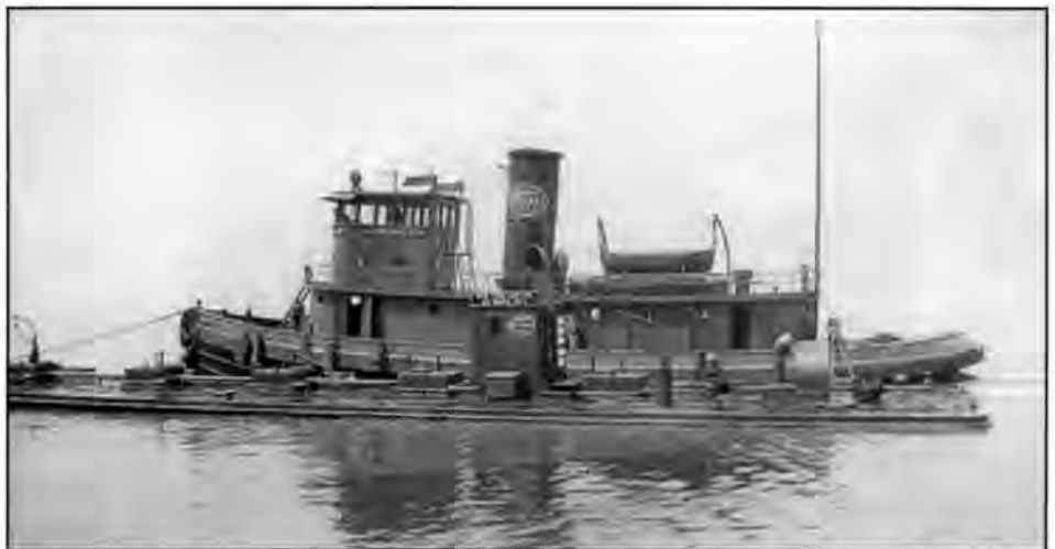
Tug No. 34 , one of the two 1926 diesel tugs, is moving the New York Central Oil Barge No. 2 in July 1934. The New York Central was an early convert to oil for generating steam for its tugboat engines, so it owned several of these very low profile oil barges. They came in handy when diesel tugs were acquired. NYCSHS collection.
