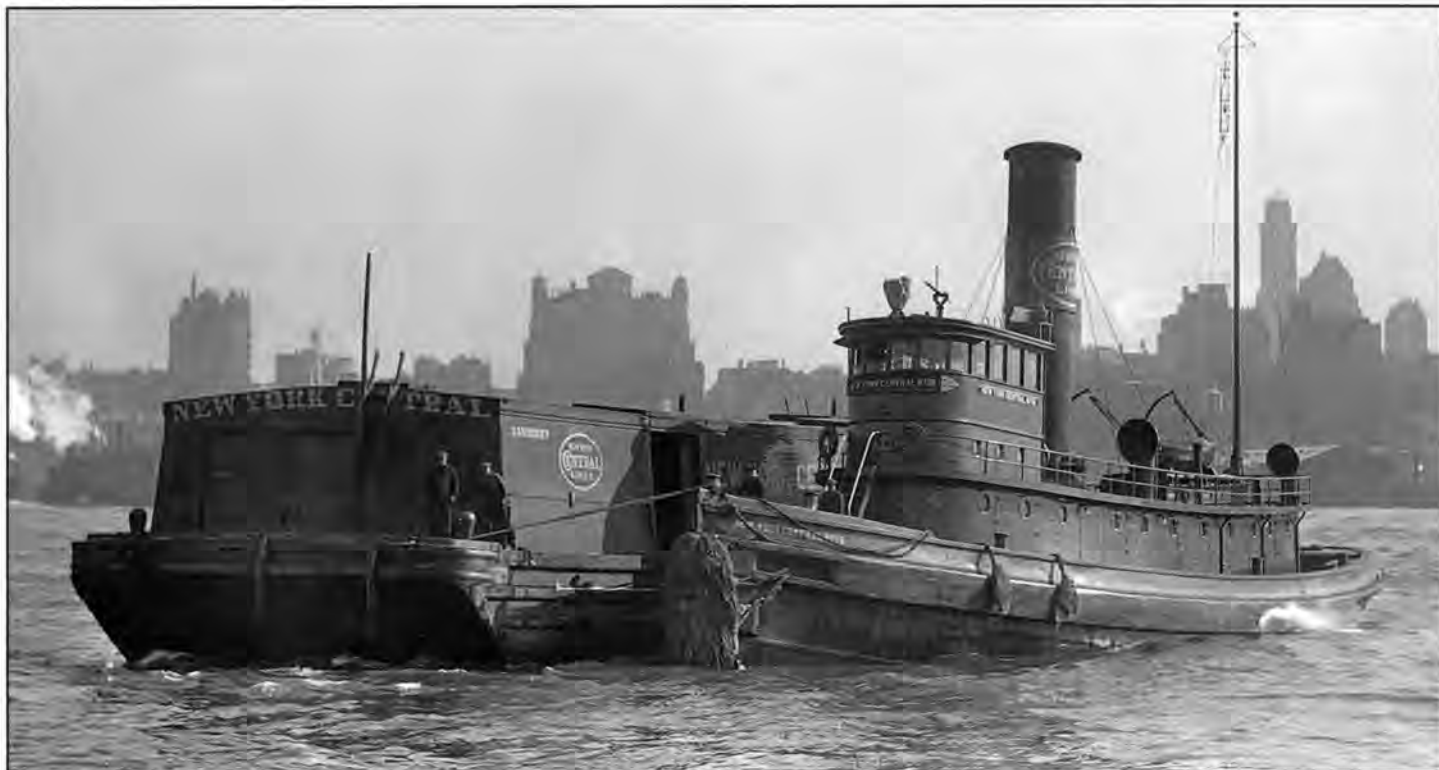
Tug No. 18 maneuvers the covered barge Sandusky in the New York Harbor. This tug was built in 1913 and was longer (111 ft.) and more powerful than the railroad's "main" boats, in fact she was the most powerful tug in New York Harbor in 1915, rated at 1087 HP, with a two-cylinder compound engine. She was built by Marvel at Newburgh, New York. In 1925 she was equipped with a new innovation: a radiotelephone! H. L. Vail/NYCSHS Collection.
