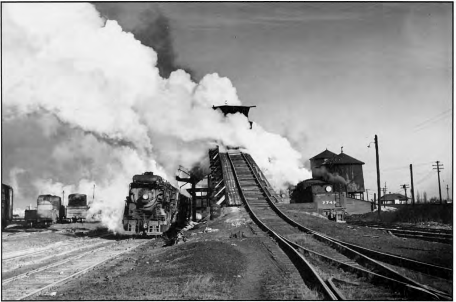
Coaling tower at Lyons Yard, Danville, Illinois on a -14 degree day in February 1949. H10b 2369 on the left, U3a 7749 on the right. Photo by Irvin Baer.
