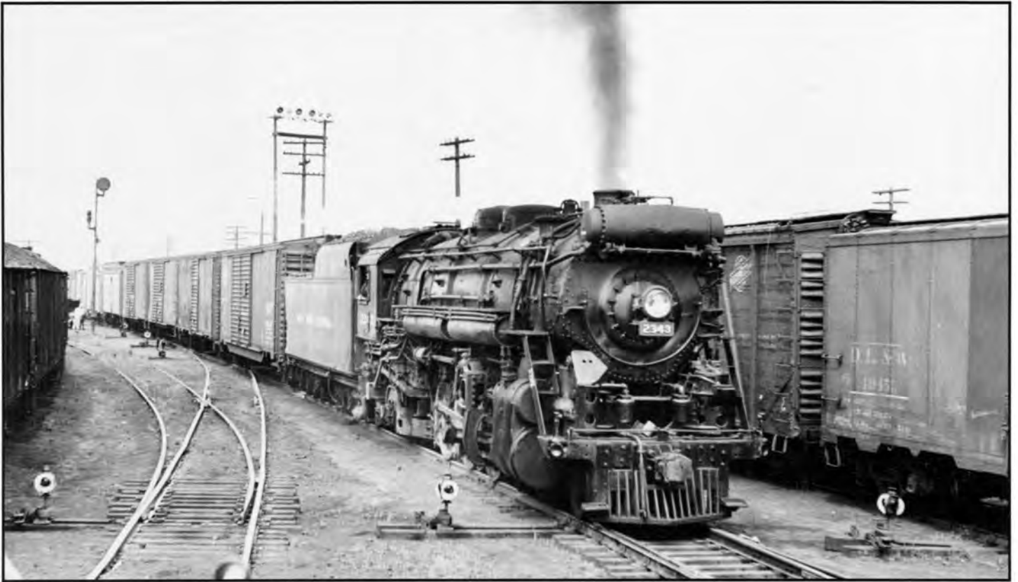
H10b 2343 at Central Ave., Detroit, Michigan, July 28, 1951.
