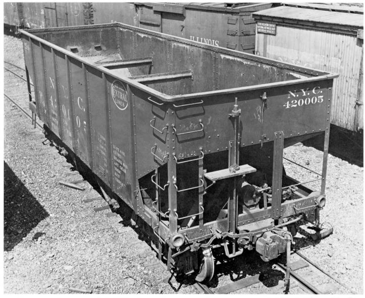
Three-quarter view of NYC 420005, Lot 378-H, shows two of the three crosstie braces used in the original USRA design, and the vertical staff lever-type hand brake. Note the brake cylinder mounted above the center sill, with cylinder head towards end of car.
