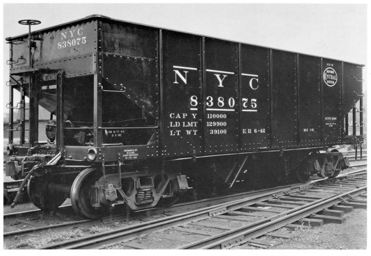
Three-quarter view of car 838075, Lot 410-H, as rebuilt at East Rochester in 1942. The original USRA side construction is retained.
