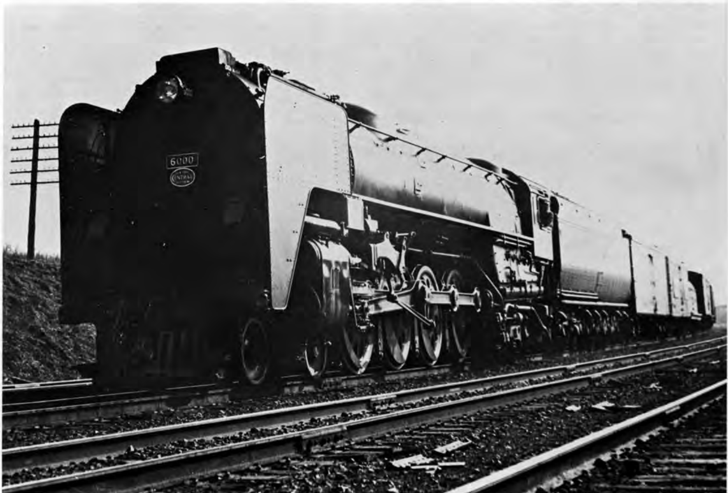
The first of the fleet, Niagara 6000 class S-1a is shown here rolling a milk train near Cold Spring, N. Y. in April, 1945, only a month after she was built at Alco's Schenectady Works. Note that 6000 is still equipped with the 75" drivers which gave her a slightly "top heavy" look that was remedied later when 79" drivers were applied.
