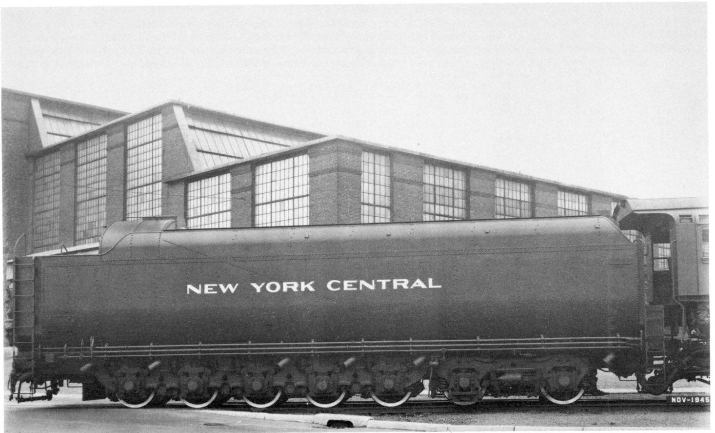
Right side of PT-5 tender built by the American Locomotive Co., November 1945. Note train control equipment compartment at rear of tender, and vent valve compartment below letter "O." Photo from Alco Historic Photo collection.
