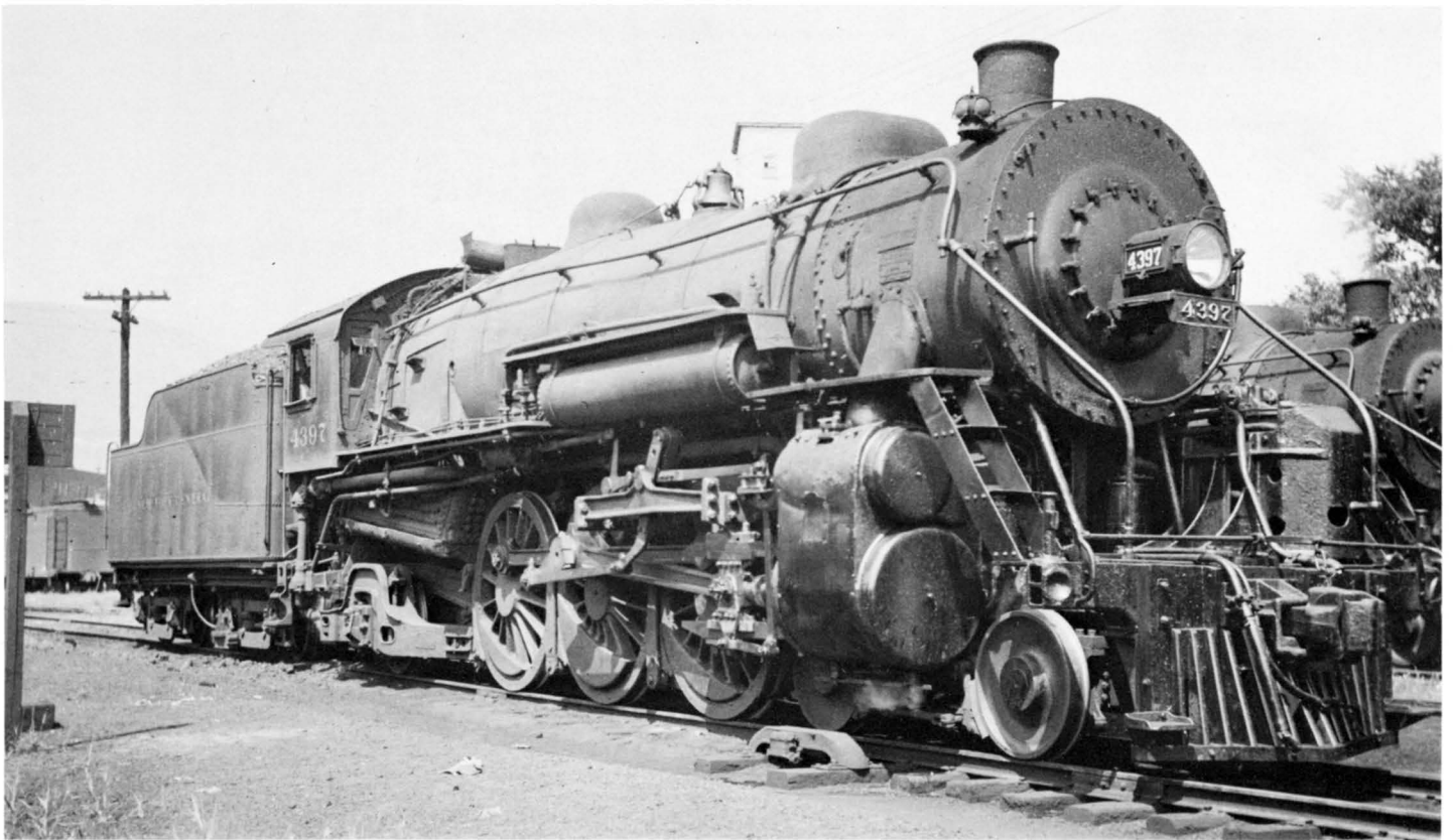
Shortly after midnight on April 12, 1925, K-11f 3183 was pulling southbound Adirondack Division No. 4 and as they were slowly crossing a new fill along Beaver River Flow, the embankment suddenly settled and the 3183 with the mail car and express car slid down into about fifteen feet of water. It took the wrecking crew several attempts to dig the 3183 out of the muck and goo. Sent to West Albany Shops, she emerged in July, 1925 as a rebuilt K-11f and later in the 1936 renumbering she received No. 4397. Here she is shown at North Adams, Mass. in August 29, 1937 while assigned to the Harlem Division.
