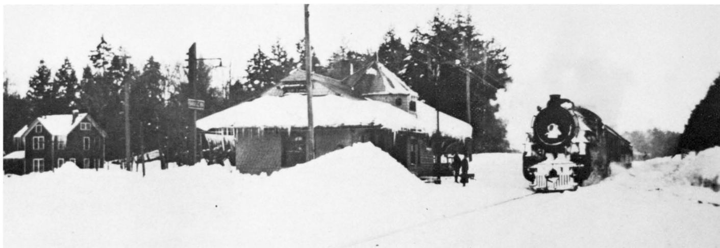
Train No. 3 with K-11a No. 4490 in command drifts into Saranac Inn for a station stop to pick up the mail, some items of express, and maybe a passenger or two and then hurry on to Malone and her terminal at Montreal on March 26, 1940.
