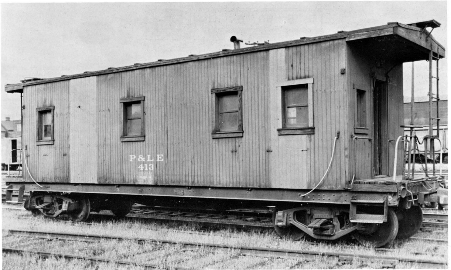
P. & L. E. #413 illustrates one type of wartime caboose used by the railroad. This box car conversion featured end platforms and stirrup type steps.
