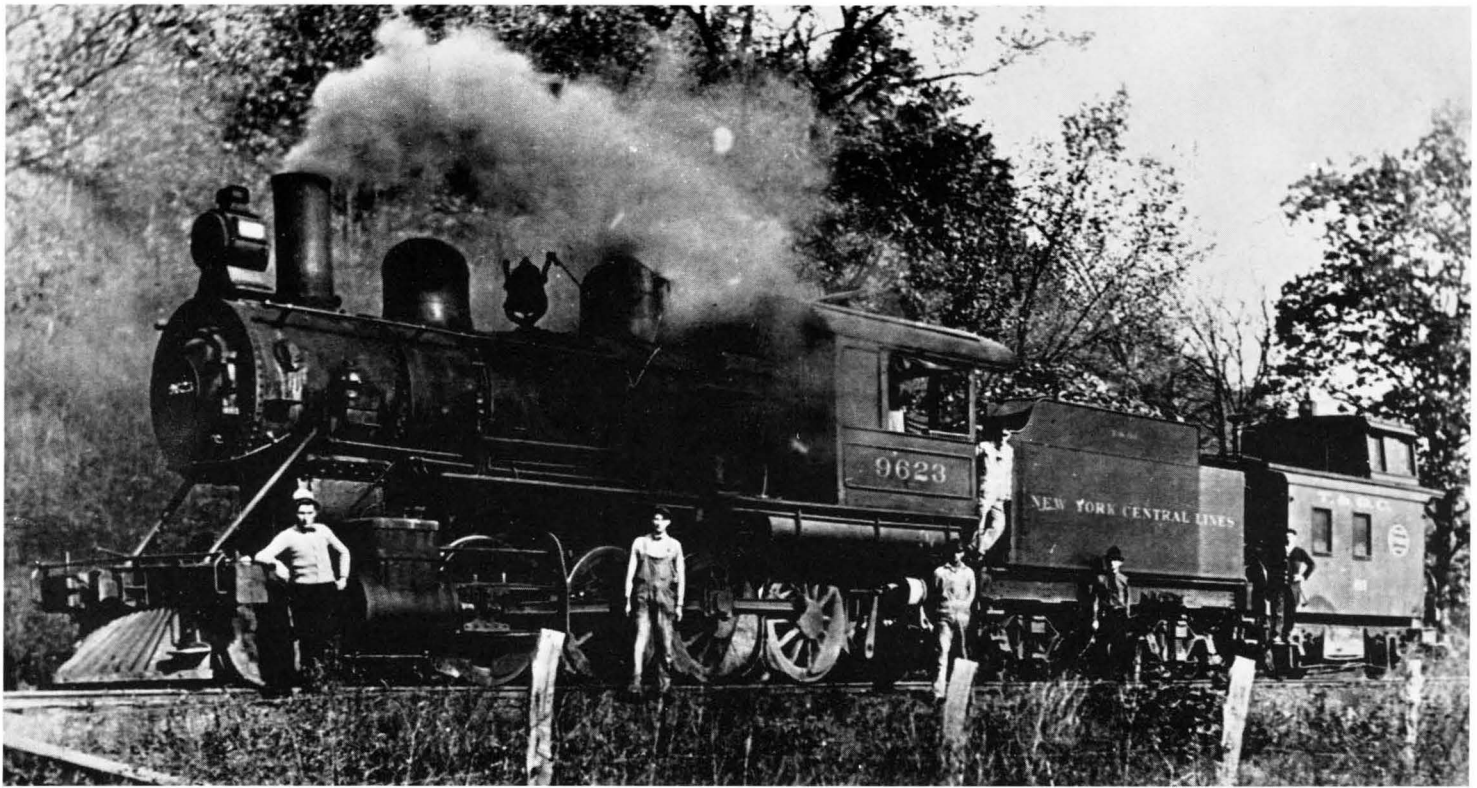
Here is another type of N. Y. C. Lines four wheel caboose, this time from the Toledo & Ohio Central. Caboose No. 61 seems to have a cupola nearly as big as it's whole body and is set well to one end. There appears to be a tool box mounted between the wheels and a marker lamp in the middle of the cupola roof. 2-8-0 9623 was built by Rogers Locomotive Works in 1903 as No. 323. This photo must have been taken after 1912 since this locomotive recieved it's new number by that time. This lanky looking class G-95A consolidation was scrapped by 1925. Coleman Collection-Ohio Historical Center - via Al Shade
