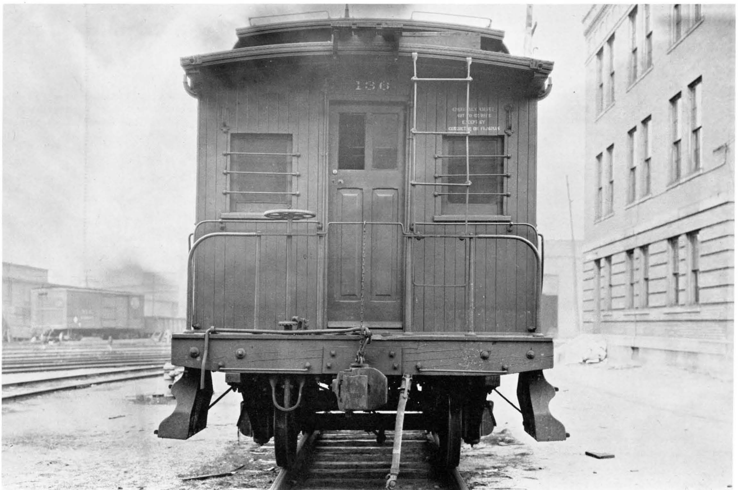
End view of Pittsburgh, McKeesport & Youghioghenny No. 136 shows paneled doors and window safety bars.
