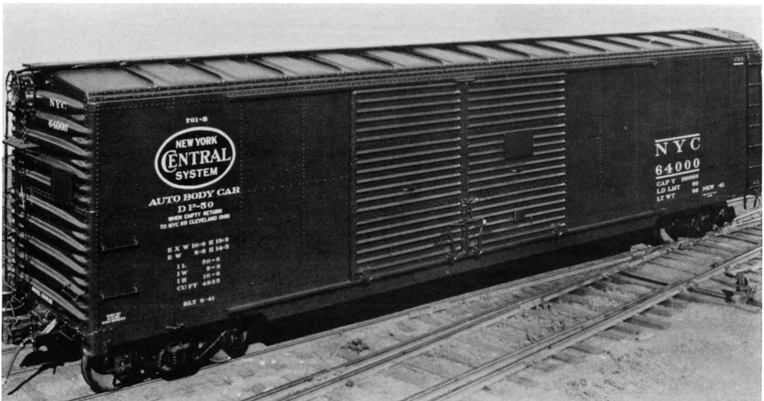
N. Y. C. 64000, 50' Auto - Box Car, Lot No. 701-B, Red Car with 48 3/8" x 32 1/2" Oval. Note once again the reversed lettering on the double door car. Stenciling on this car indicates that it was used to transport auto bodies, probably for the Fisher Body plant in Cleveland, Ohio.
