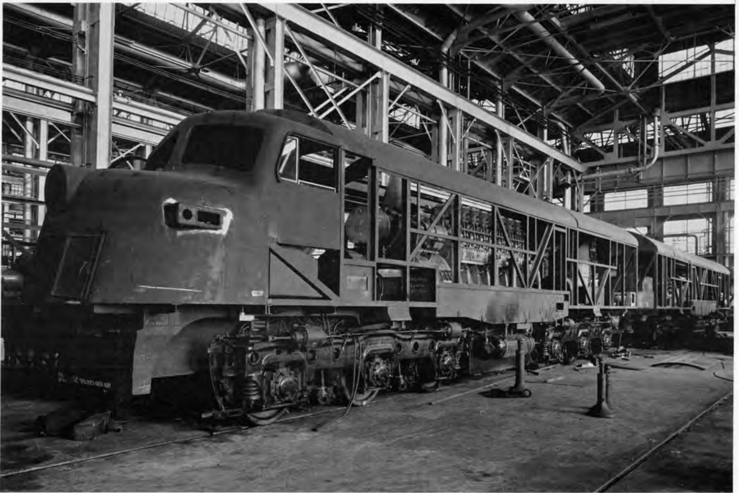
N. Y. C. DCA "Combination" diesels under construction at Baldwin Locomotive Works in 1947. Note massive cast steel underframe and heavy girder carbody construction. Known to "Central" employees as "Gravel Girtys" or "Humpbacks" these locomotives were disliked by engine crews and shop forces wherever they operated. The Baldwin 608 SC eight cylinder engines were replaced with EMD 567C V-16 power by the N. Y. C. at the Collinwood Diesel Locomotive Shop in 1955 in an attempt to cure some of the problems. The operation was not a success. Diagram on page 68.
