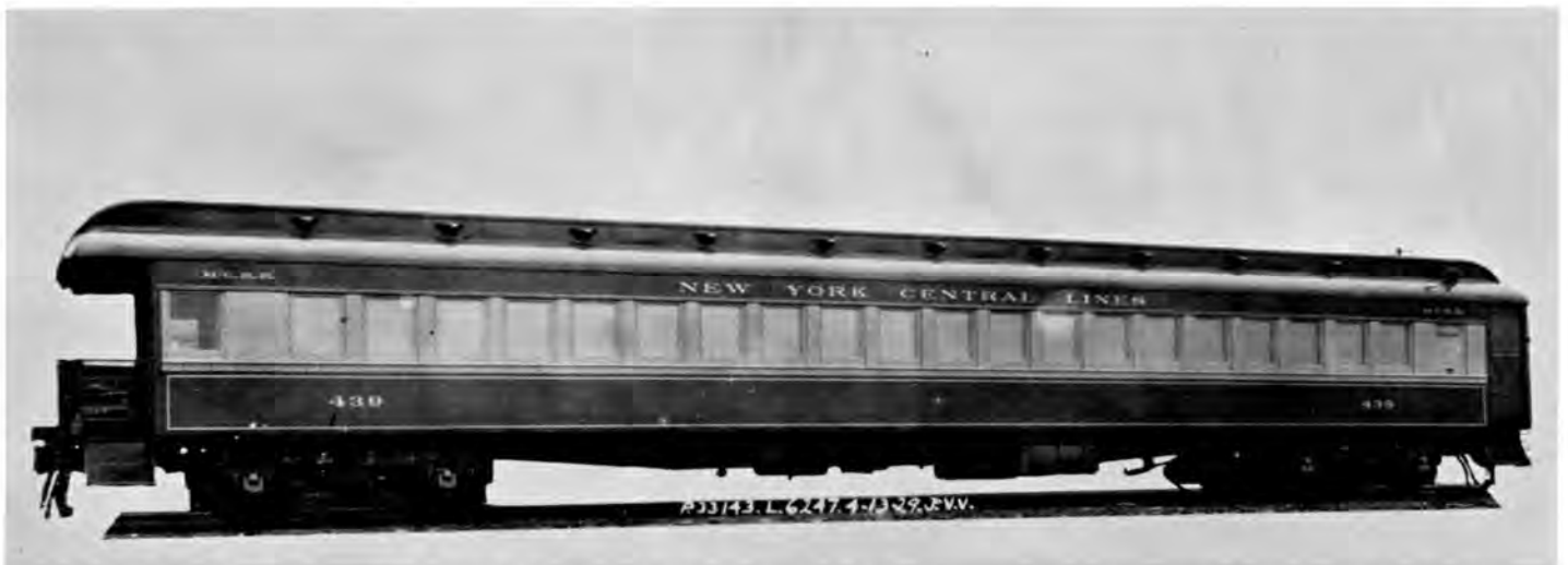
N.Y.C.L. (M.C.R.R.) observation 439 as rebuilt from coach by Pullman in 1929. This car was converted back to a standard coach by Beech Grove (Indiana) Shops in 1942. Paint scheme on car appears to be "brown and fawn" as mentioned in text. George E. Votava Collection
