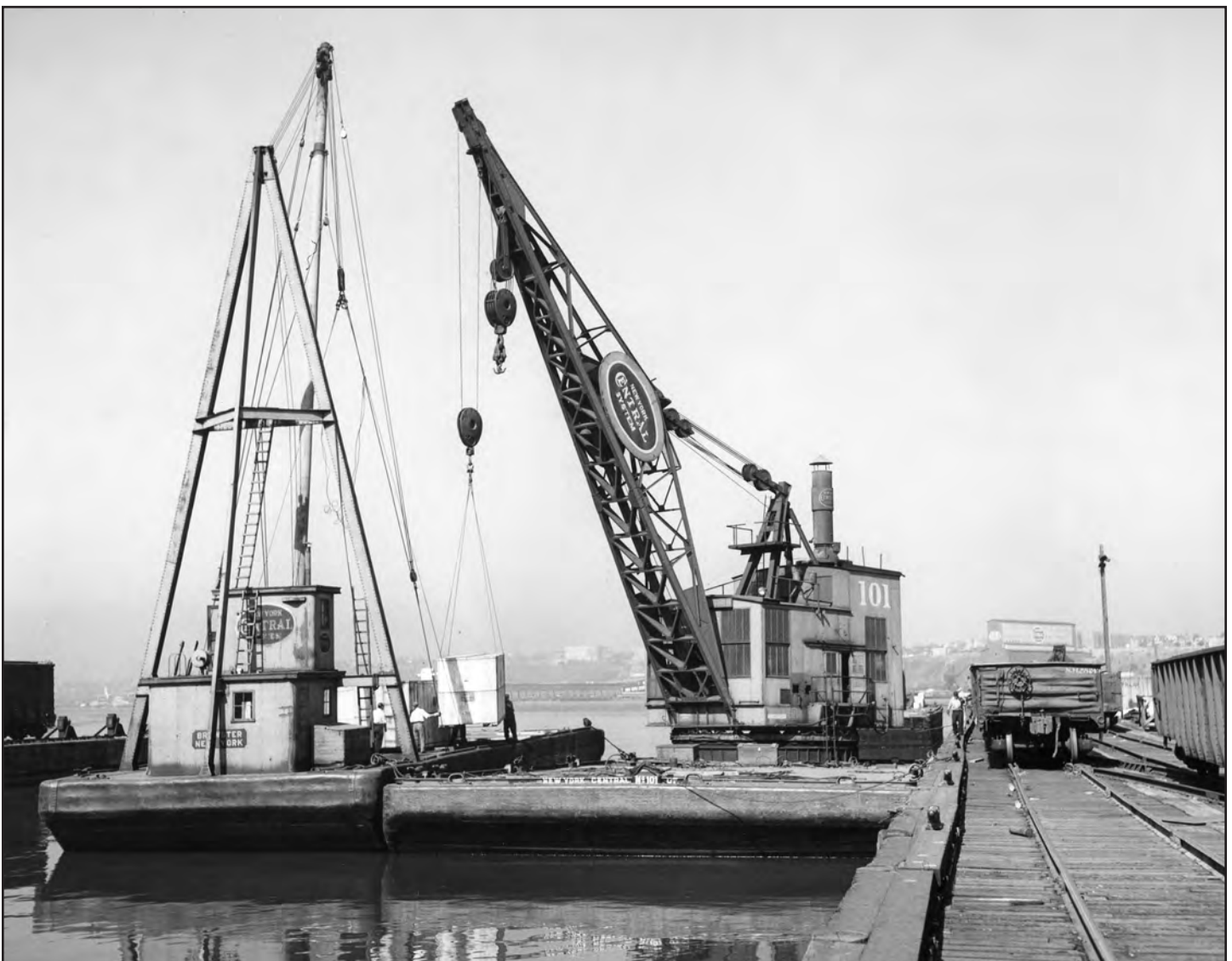
At Pier I (letter I, not number 1) in the 60th Street Yard in Manhattan, floating crane 101 (built in 1931) swings a big box from a gondola on the pier to the gasoline hoisting barge Brewster . It is not obvious why No. 101 is needed here; Brewster should be able to handle any box weighing five tons or less on its own. Perhaps the photo was staged. Both 101 and Brewster were called “unpowered craft” because neither could propel itself around the harbor; they were moved by tugs. But they did have engines – No. 101's crane was steam powered, and that of the Brewster was powered by gasoline. New York Central photo, T. Flagg Collection.
