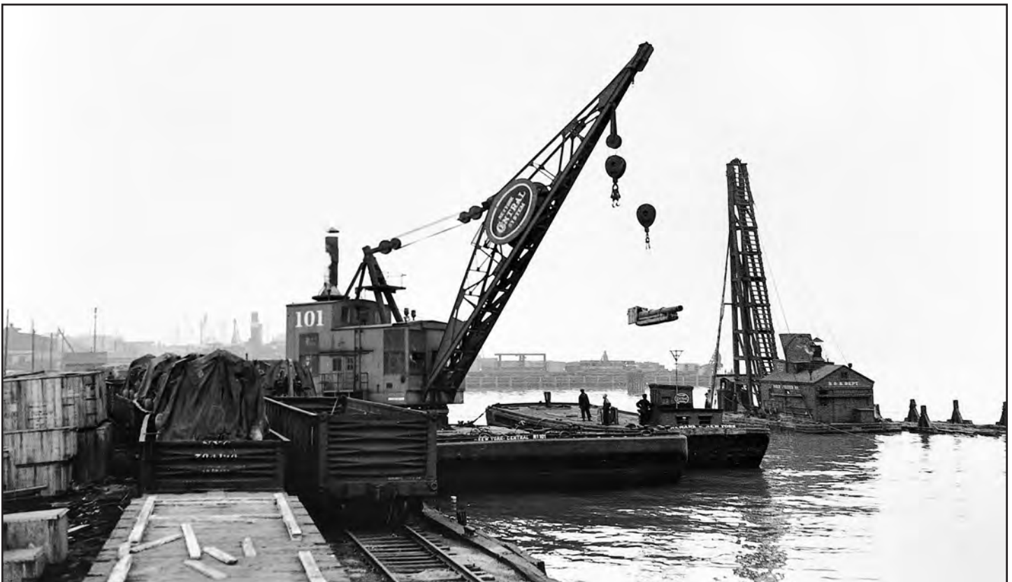
Here's floating crane 101 again, this time at Weehawken, transferring a load from a gondola to the open deck scow Newark. A veteran of about 45 years of service when this photo was taken on April 25, 1946, the Newark was built in 1900 and will survive until 1952. One of New York Central's floating pile drivers appears in the background. NYC Negative 7282-3, NYCSHS Collection.
