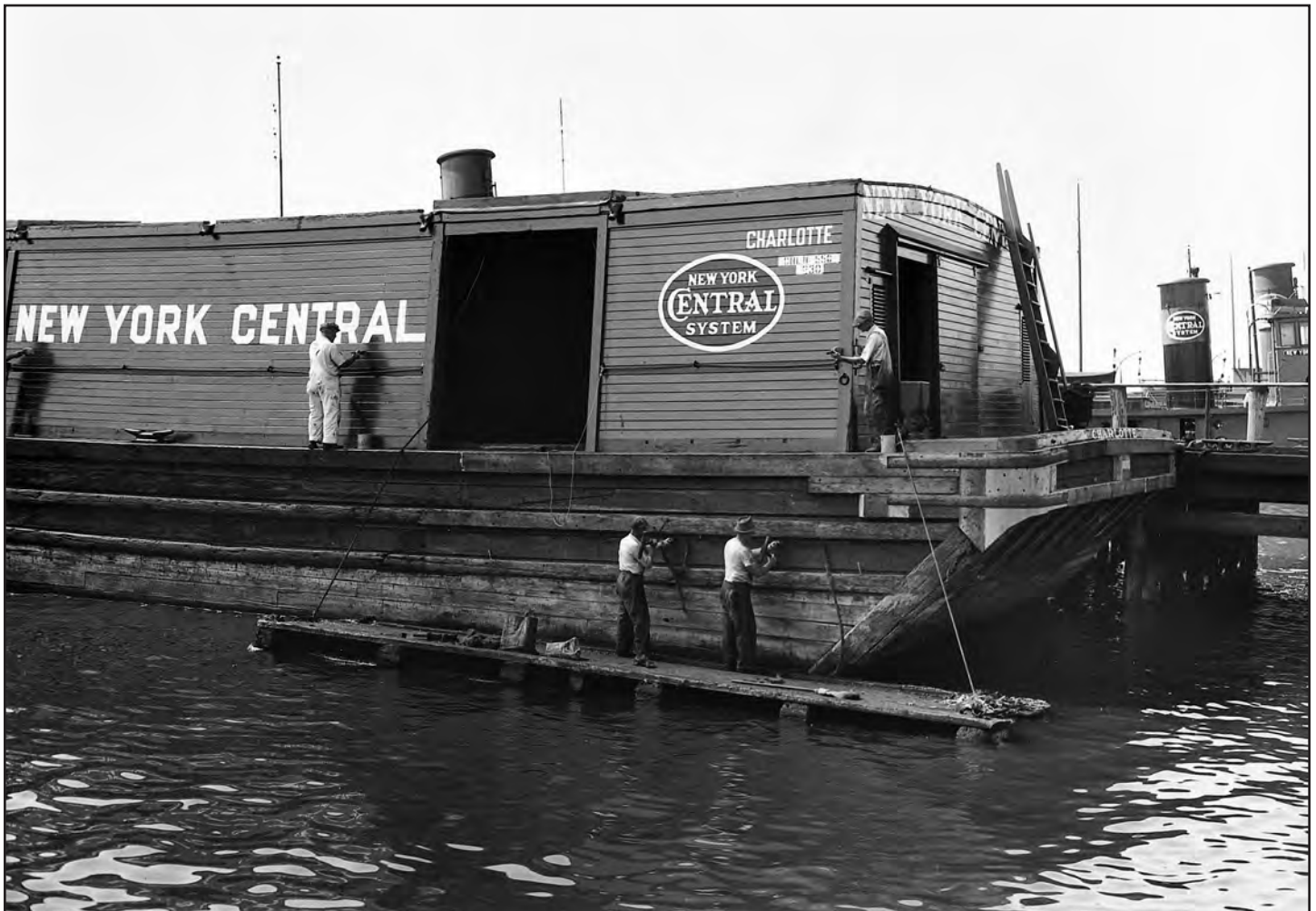
Workers at New York Central's Weehawken Marine Shop caulk and paint the wooden covered barge Charlotte on July 21, 1950. NYC Negative 9158-3, NYCSHS Collection.
