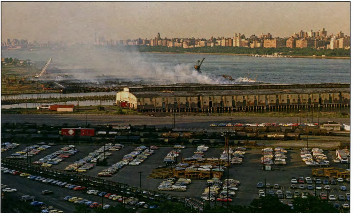
Here we see the landward end of Pier 2, still in some use in June 1976, a month after the startup of Conrail; note the freight car halfway in. A major fire the day before took out Piers 4 and 5, and a fireboat is still pouring water on the remains. The terminal is still in use for auto delivery and chemicals, but no longer handles any harbor craft. Photo by T. Flagg.
