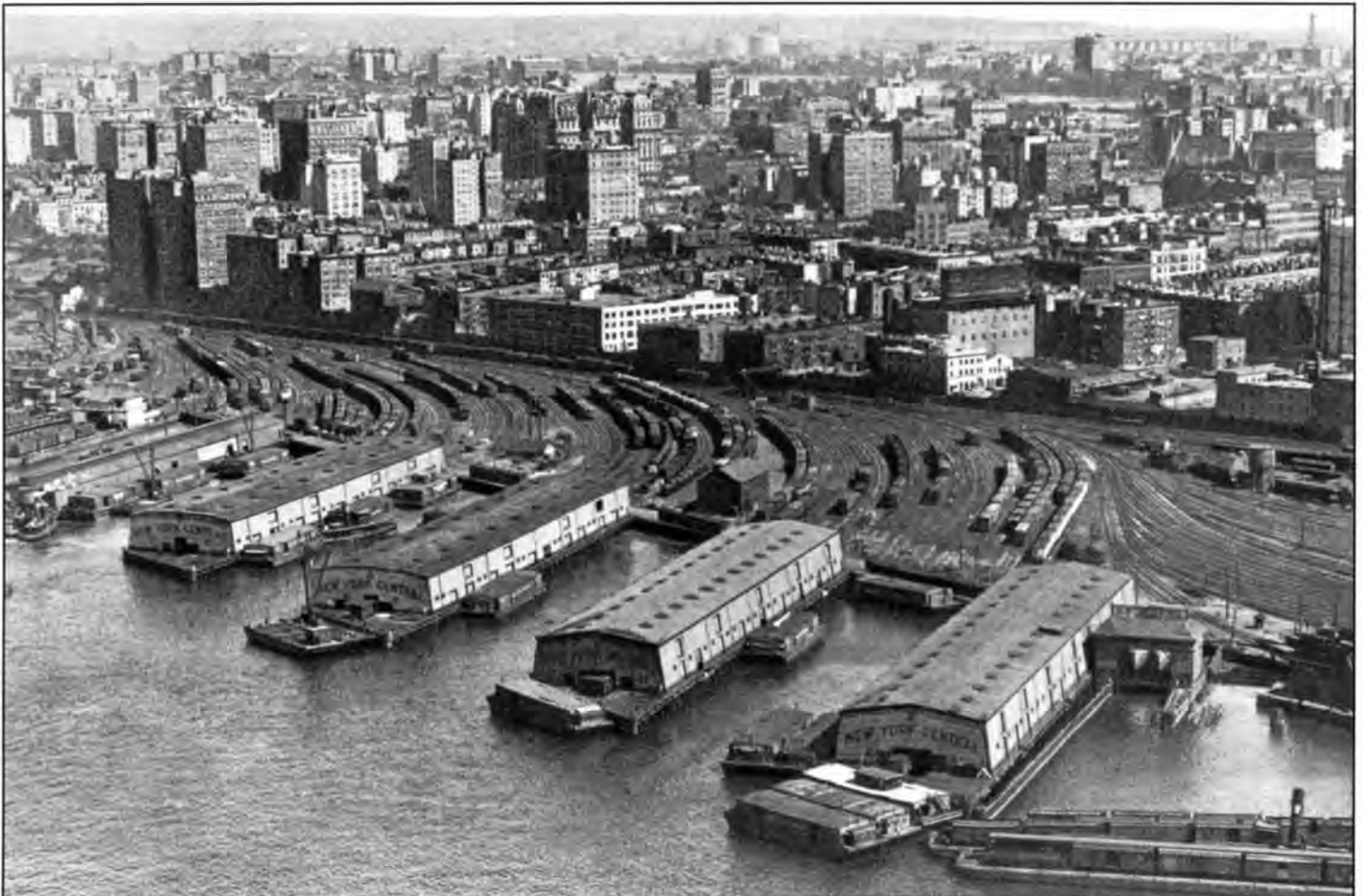
Here is a view of New York Central's 60th Street Terminal waterfront as it appeared in 1926, before the Miller Elevated (West Side) Highway was built over it in the 1930's. The rightmost pier is Pier B, with a float bridge just to the right (south) of it. That float bridge was installed about 1906 and lasted until 1956. The main three float bridges are just visible at far left. This early aerial photo appeared in a commemorative book, The One Hundredth Anniversary 1826 - April 17 - 1926 of The New York Central Railroad , issued by the railroad. T. Flagg Collection.
