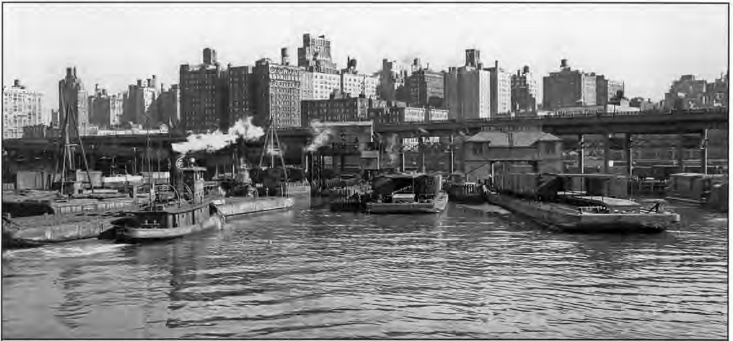
Marine operations in New York Harbor received considerable attention from the company photographer. In this 1950's photograph by Ed Nowak, the float bridges at the 60th Street Terminal are seen from the river. Station floats, with platforms between the tracks, are moored at float bridges 2 and 3, and the tug appears to be moving an interchange float into bridge 4. Pier 1, with several open barges parked around it, is on the left. The West Side Elevated Highway now soars above the length of the yard. T. Flagg Collection.
