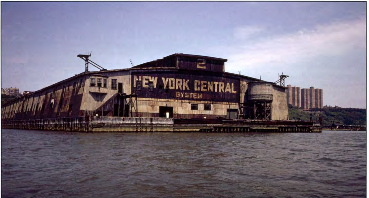
Here's Pier 2 at Weehawken again (see the photo of the same pier on page 17), now in 1977, after the elimination of the Marine Department. The railroad-style water tower for tugs shows to good advantage but, alas, there are no more tugs. Photo by T. Flagg.
