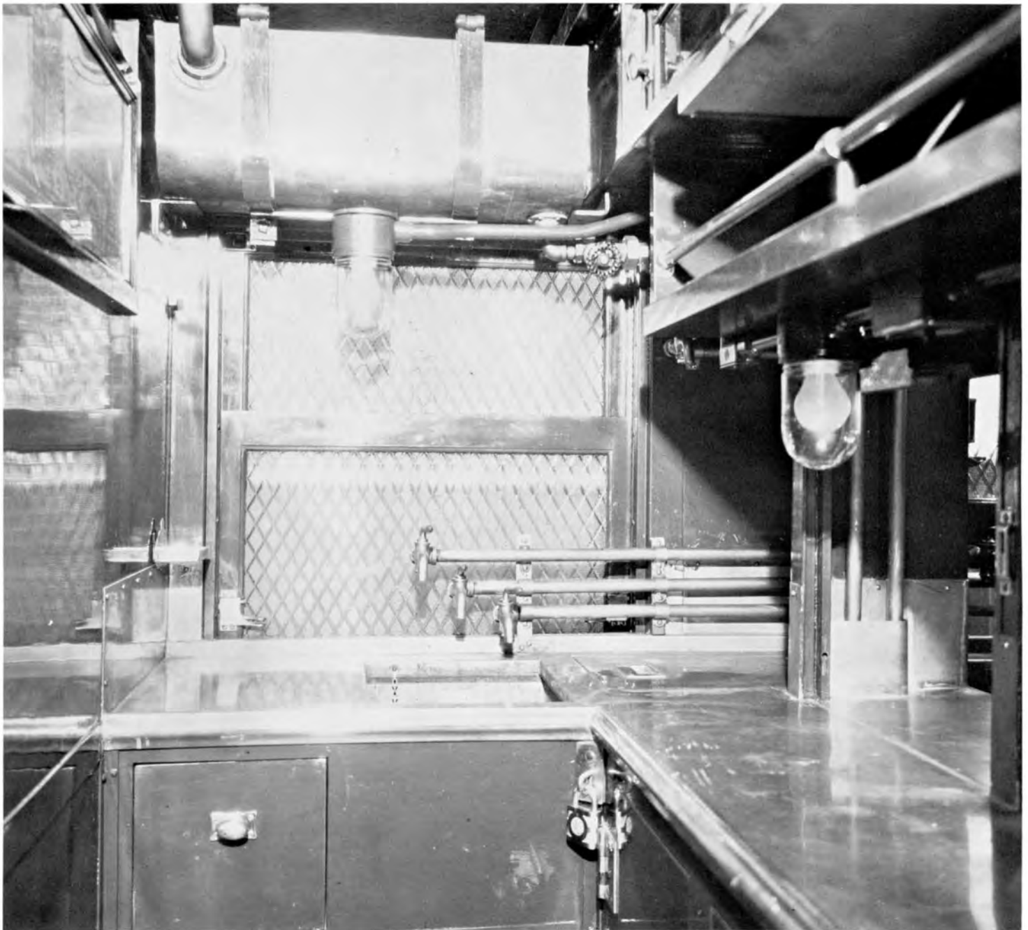
Interior view of P. & L.E. No. 99 showing one end of the pantry. Note overhead water tank and large padlock on supply cabinets below sink.
