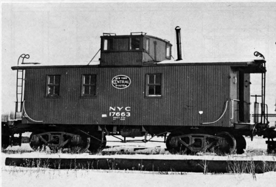
Caboose #17663 appears to be in good shape in this photo taken in January, 1963. Note the fancy "curl" on the ladder handrails which was always a distinct spotting feature of the Big Four cabooses. One of the side windows has been "planked over". Si Herring Photo
